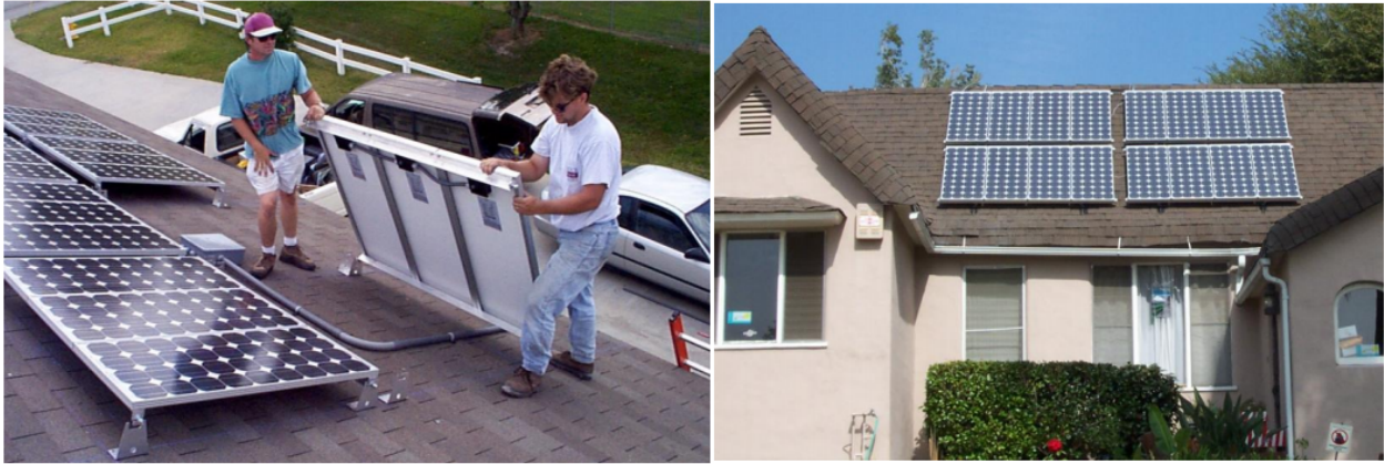
PV Installation on Roof
