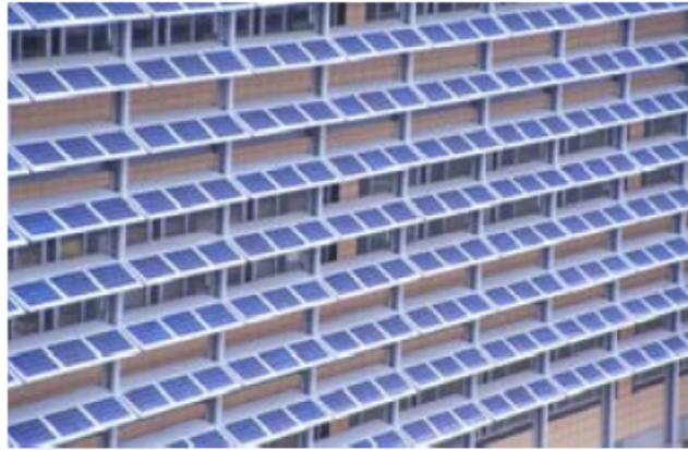
PV as Shading Device
