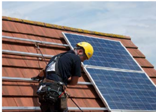
Sloped Roof PV Mounting Arrangement
